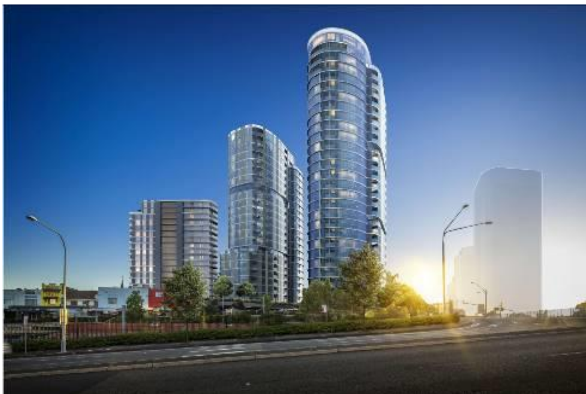
Figure 6. Photomontage of proposal as viewed from Beecroft and Epping Road looking north east.
