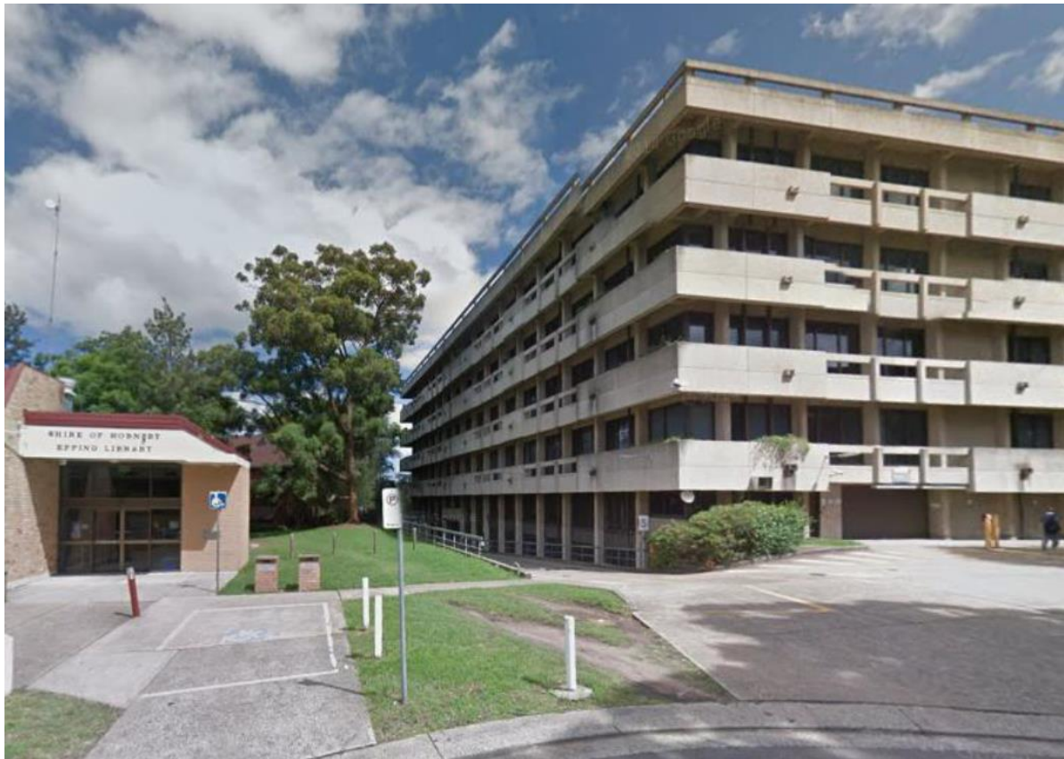
Figure 5. Existing built form looking south from Chambers Court, adjacent to Epping Library site
